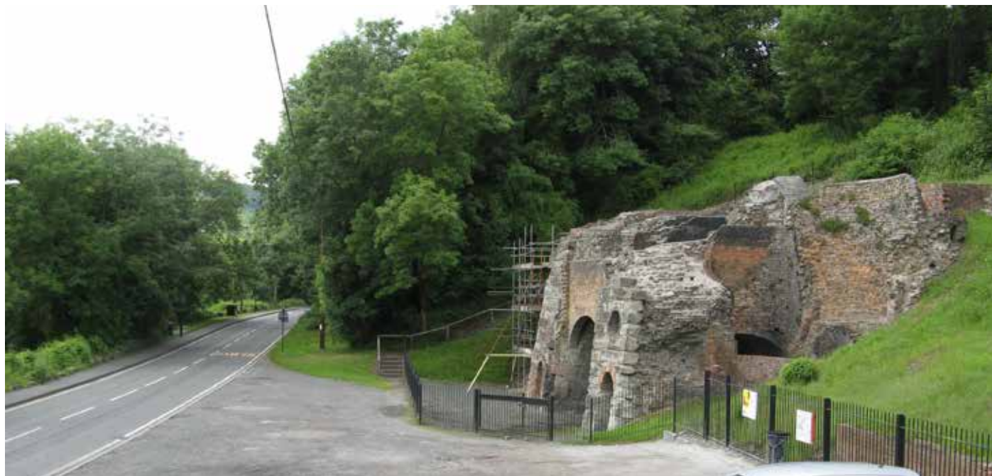
Figure 1. Bedlam (Lower) Furnace: the conserved, officially interpreted SAM. Looking west towards the Upper Furnace at Lake Head. One may compare this view with William Pickett's aquatint: 'Iron work, colebrook dale'. Pickett's two chimneys, locating the Upper Furnace, stood centre-left – where Waterloo Street bends to the right.
