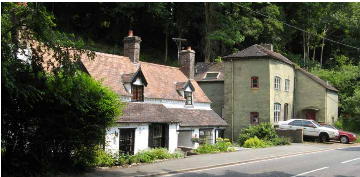
Figure 3. Bedlam Upper Furnace: An atmospheric steam engine house (c.1757) standing intact to the rear of 11, Waterloo Street, Ironbridge.
