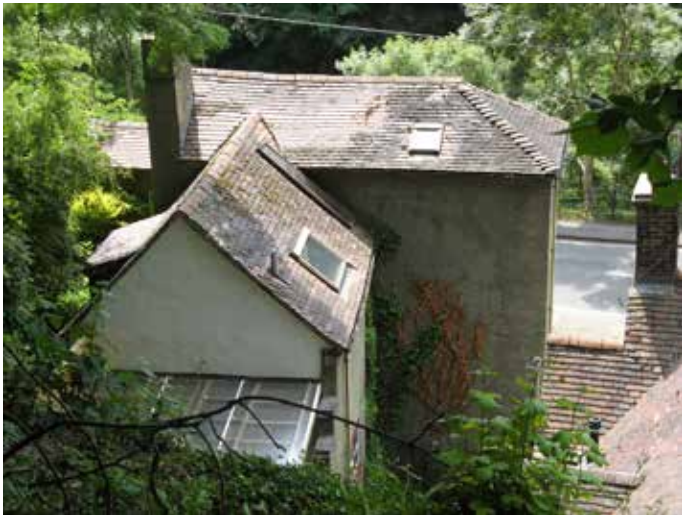
Figure 2. Bedlam Upper Furnace: The Lake Head cottages, 9, 10, & 11, Waterloo Street, Ironbridge. These dwellings were adaptively converted from the Upper Furnace atmospheric steam engine house (built c.1757); the smithy (built c.1758); and the joiners' shop (built c.1770-76). Compare these buildings with the Bedlam Furnace buildings as depicted by P.J. de Louthembourg in 'Coalbrookdale by Night'. Note: the hip-roofed building and lean-to, centre-right, are later additions.
