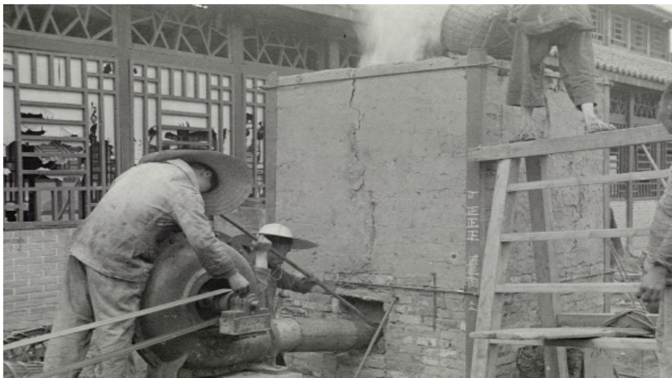
Fig. 1 Men at work at a cupola furnace in the Central Machine Works in Chengdu, SW China, May 1943 (Photograph: Joseph Needham).
