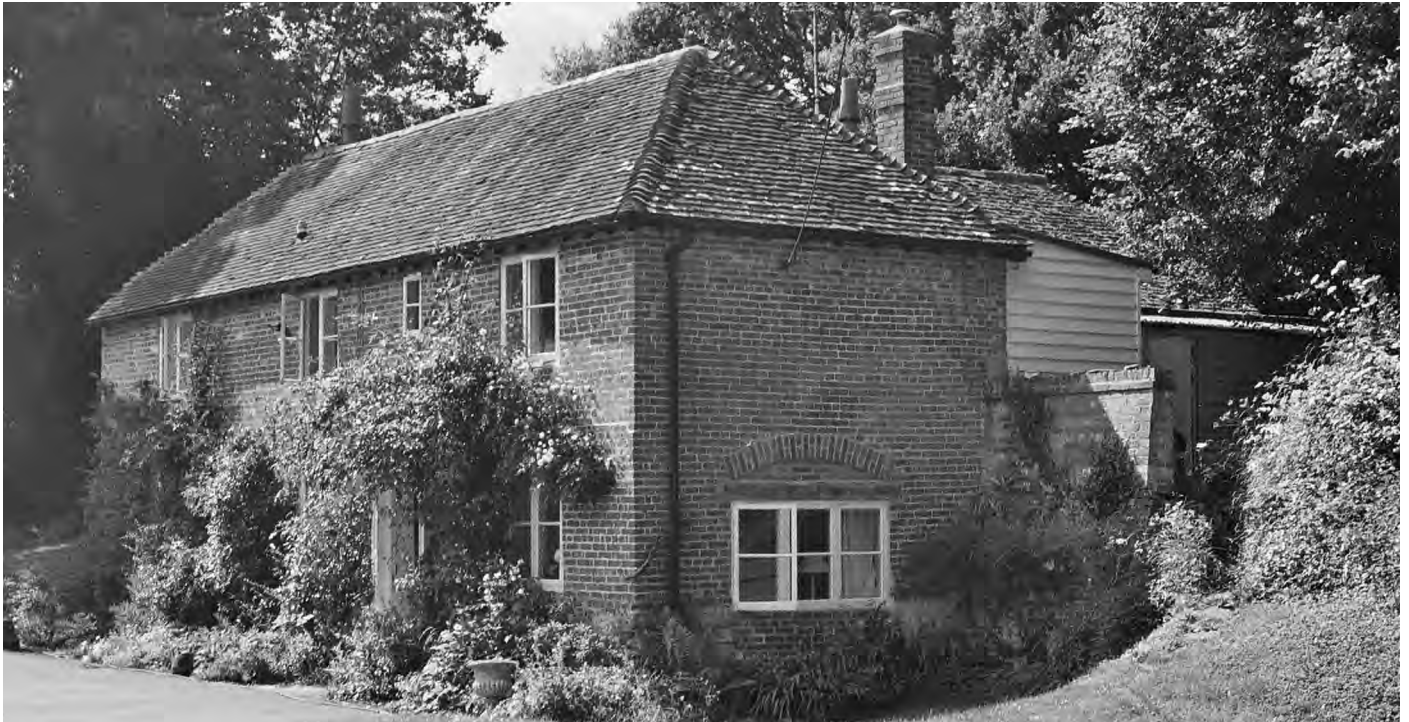
The furnace house at Ashburnham, Sussex - probably originally built as part of the boring mill.
