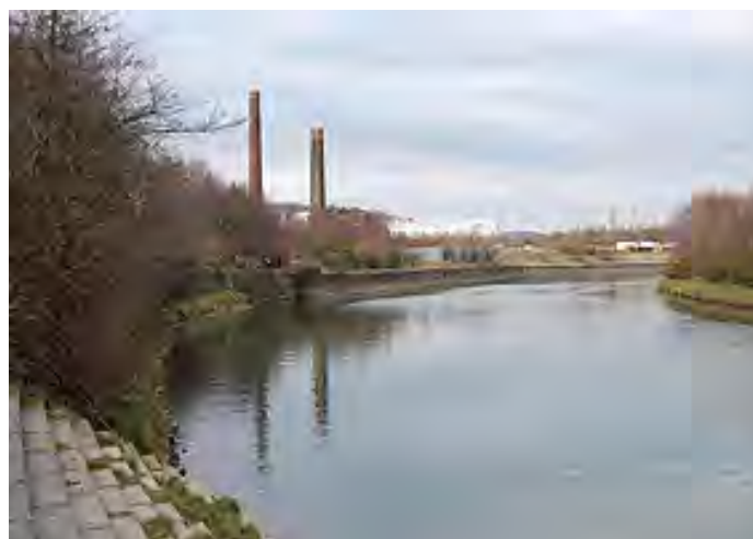
The riverside at the Hafod Copper Works.
