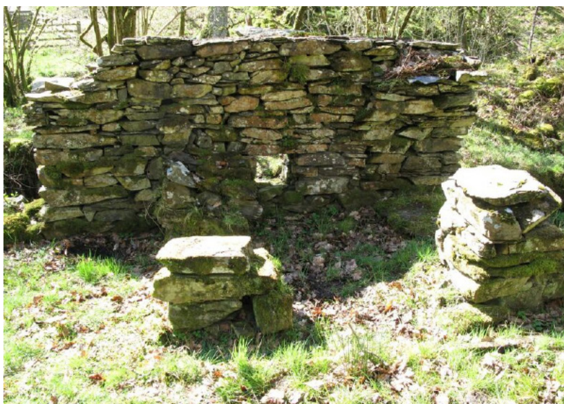
Fig 1: The hole in the back wall of the hearth, tuyere entry from left
