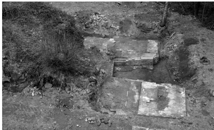
Figure Two. Stirchley furnaces: view of the southern furnace during excavation showing the outline of the furnace bases.
