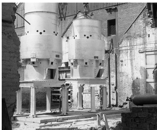
Figure 3: Erection of New Cupolas
