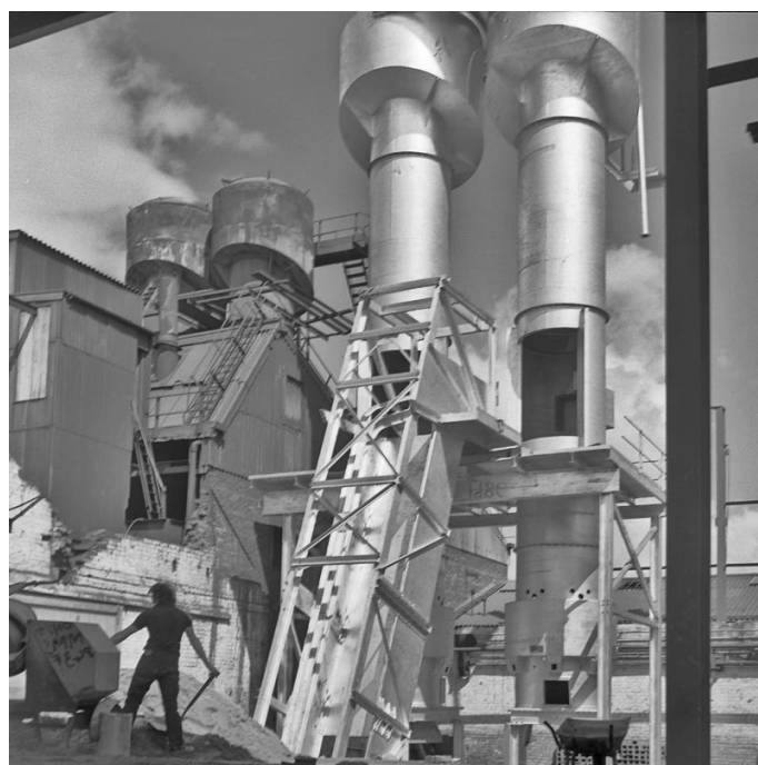
Figure 2: Erection of New Cupolas
