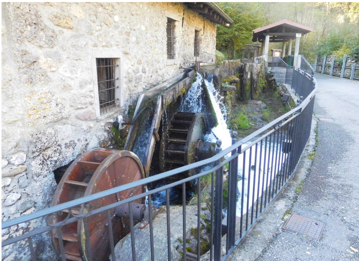
Fig.3. The two waterwheels in the foreground and the trompettes are visible slightly further upstream
