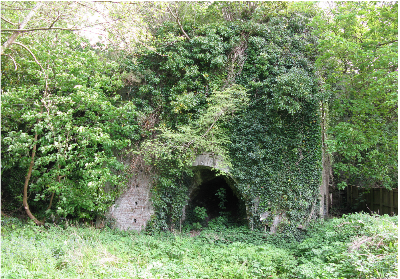
Fig.1. Alexander Raby's furnace today at Llanelli, South Wales
