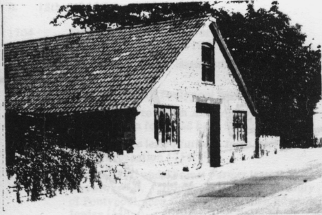
F Abbey (Lower) Forge/Corn-mill building at Tintern, west face.
