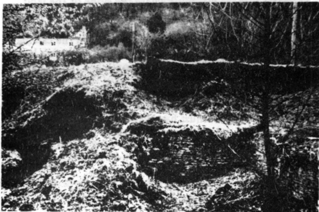
B General view over blast furnace site, showing interior of furnace on left and wheel pit and blowing house in right foreground.
