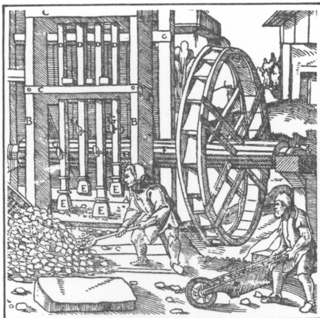
Crushing copper ore with stamps. Agricola Book VIII
