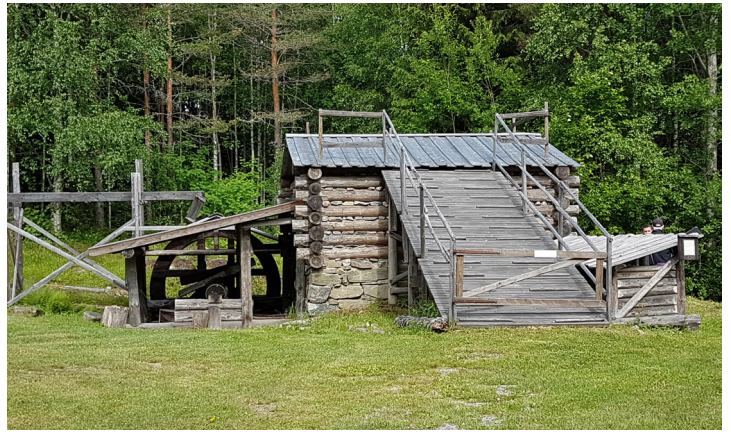
Figure 4: The replica furnace at New Laphyttan (with a temporary roof); the waterwheel driving the bellows is to the left and the charging ramp in front.
