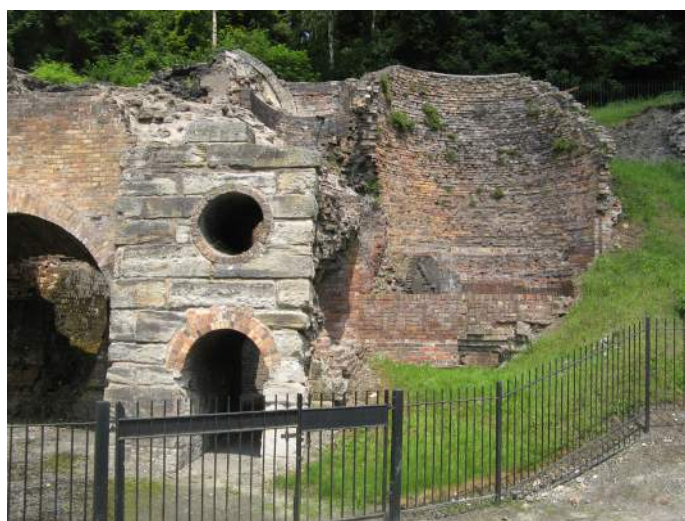
Bedlam “Furnace II” – right. The standing remains of the cone-like furnace structure.
