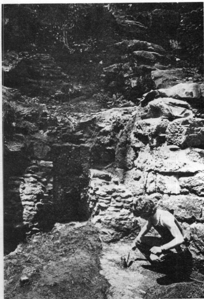
Figure 6 View of the forehearth area. The black, raised mass leading from the tap hole (middle ground) out into the casting floor (foreground) is a shadrach or salamander (composed of cast iron, slag, ore, and charcoal bits) representing the Eaton's last cast. It plugs the tap hole and rises more than 60 cm into the crucible.
