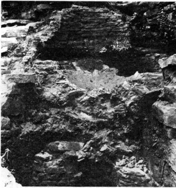
Figure 2 Bosh area of the Eaton Furnace showing inturned bosh and section of inner chimney lining of refractory sandstone. The debris in the centre is the collapsed insulating layer material. The top of the tap hole is visible in the middle foreground.
