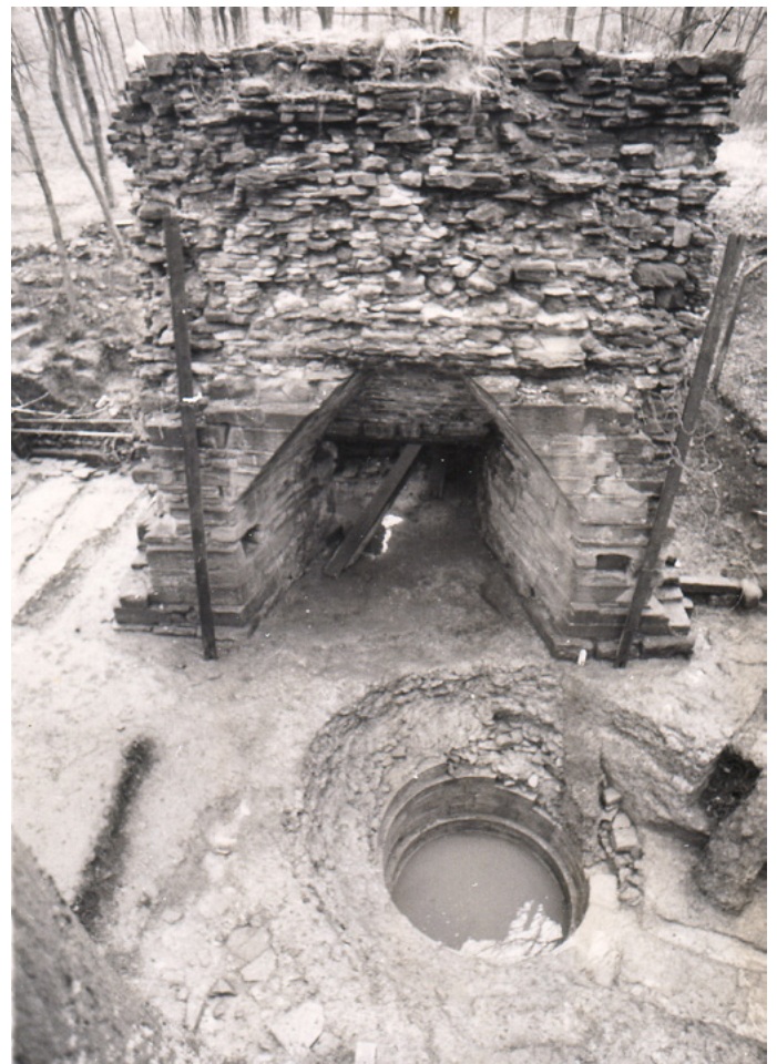
Rockley blast furnace c. 1700 during excavations in the 1980s by David Crossley (note casting pit in foreground). Rockley is located close to junct 36 M1 north of Sheffield.
