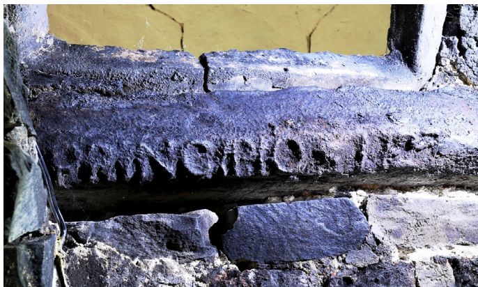
Cast iron pig in situ forming lintel to oven.
