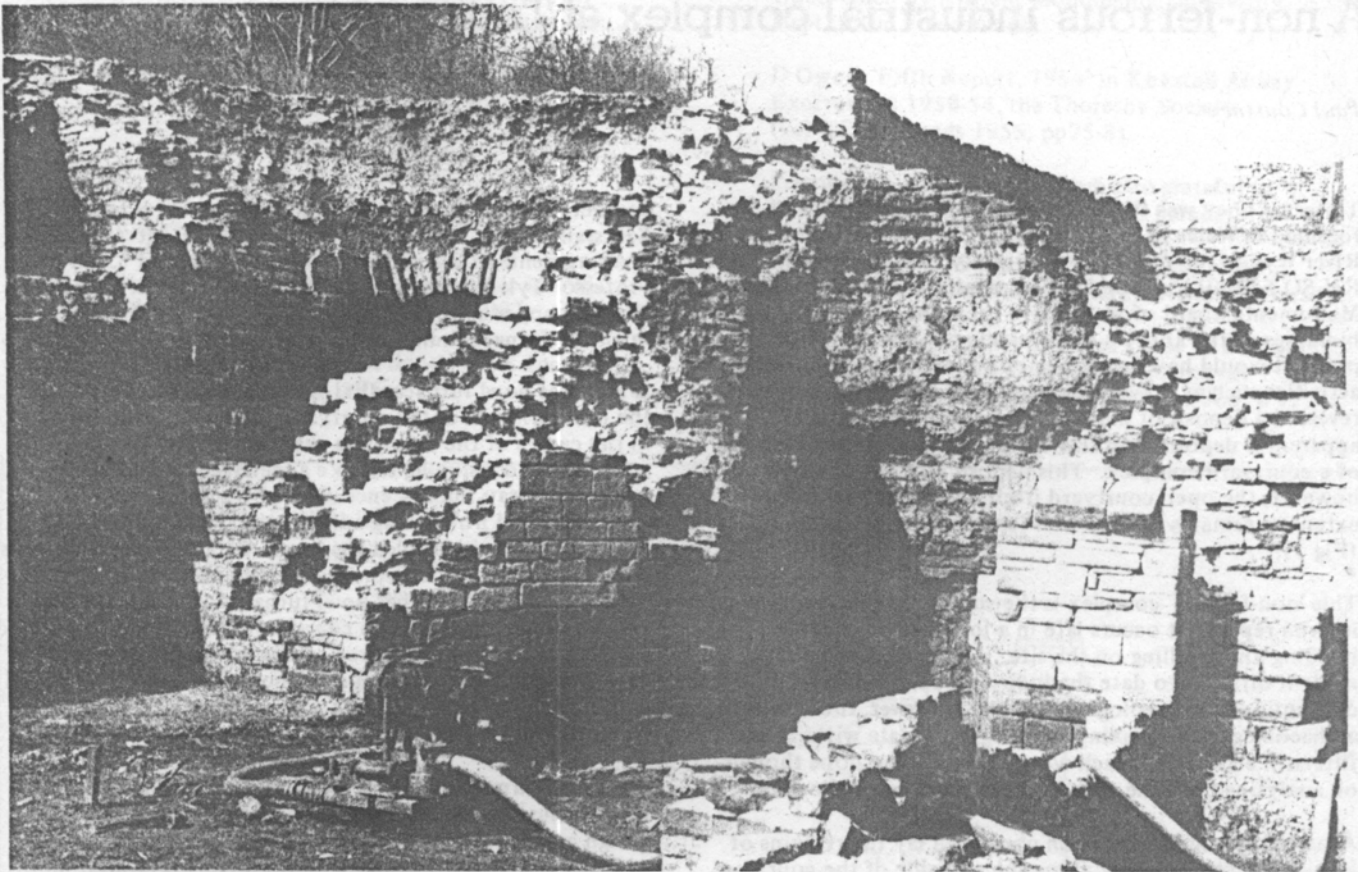
Fig 14 East face of furnace with charging platform above (picture, Gwent County Council)
