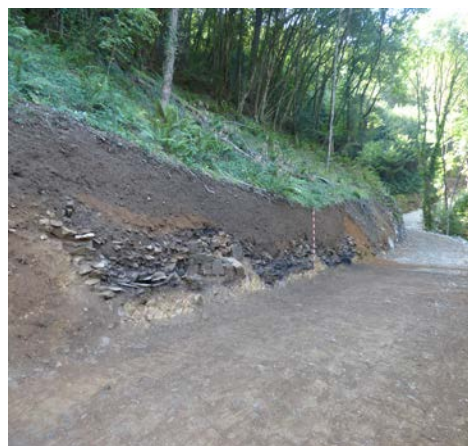
Fig. 2. Section of As Mestas discovered after the clearing of the road
