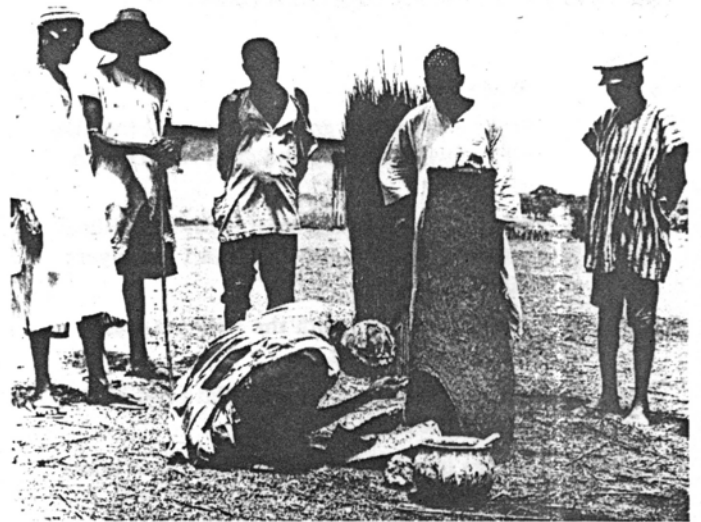
Fig 8 Cutting out the hole for the tuyere.
