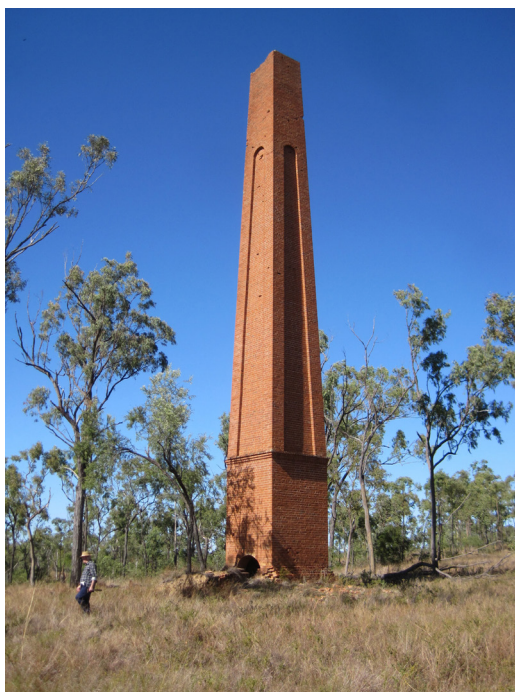
Figure 3. The smelter chimney at Argentine
