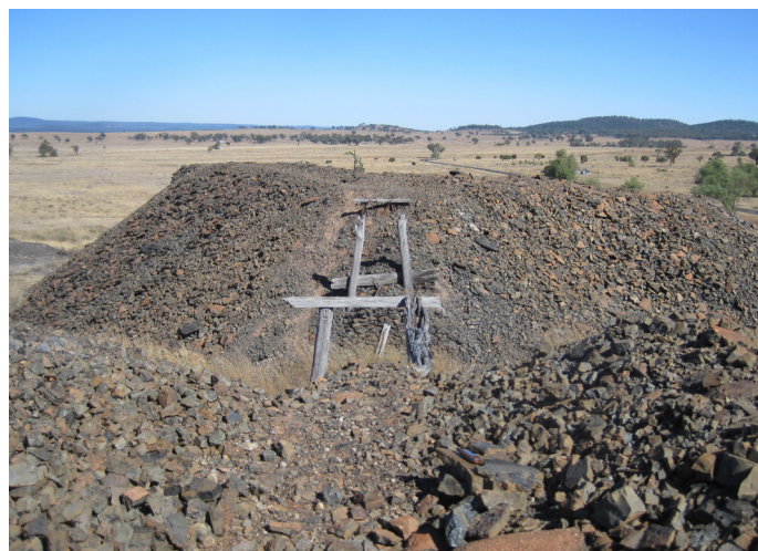
Figure 5. The remote slag dump with remains of tramway bridge, at Silver Spur.
