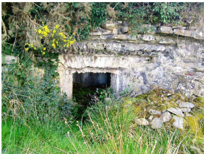
Derryoover Blast-Furnace. One of the two lower level 1.5m square exit ports with rear wall just visible at the back
