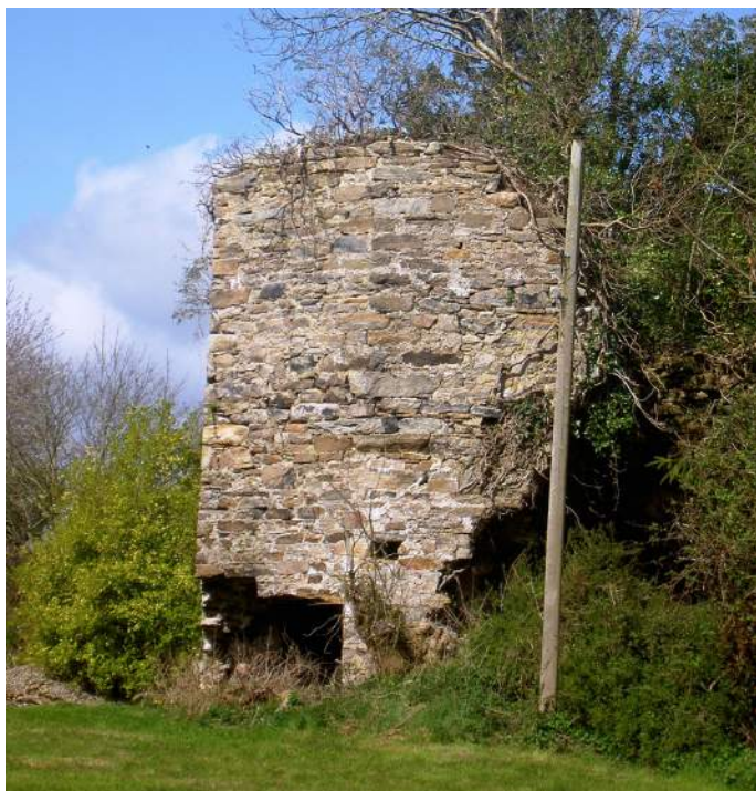
Whitegate Blast-Furnace Tunnel Exit
