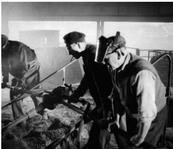
'Men of Corby' tapping a blast furnace
