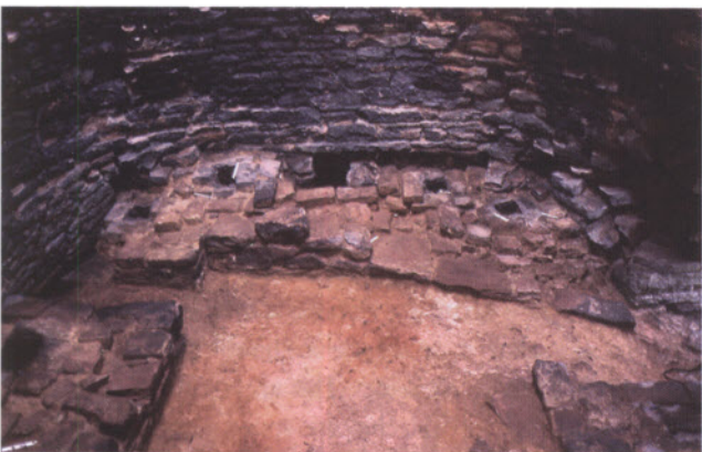
Figure 87: The interior of the cone of the cementation furnace at Derwentcote showing many internal flues (square holes) rising from the firing chamber beneath.
