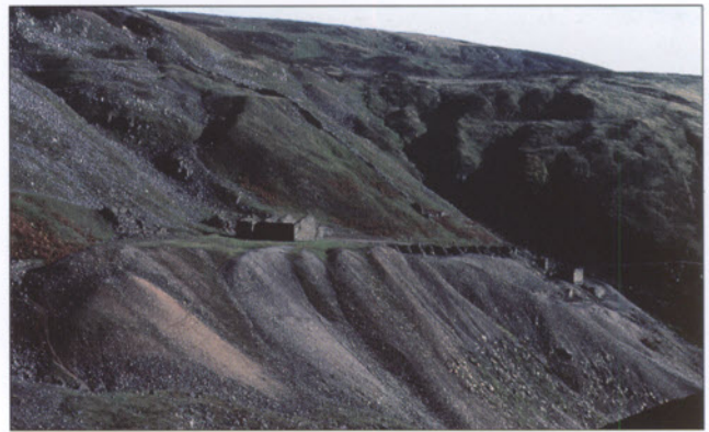
Figure 35: Gunnerside Gill, North Yorkshire: the surface of a lead mining landscape. Virtually the whole surface on both sides of the valley and on the high moorland beyond is occupied by a palimpsest of hushes, shafts, levels, ore-dressing floors, and their associated waste tips, water supplies and transport networks.
