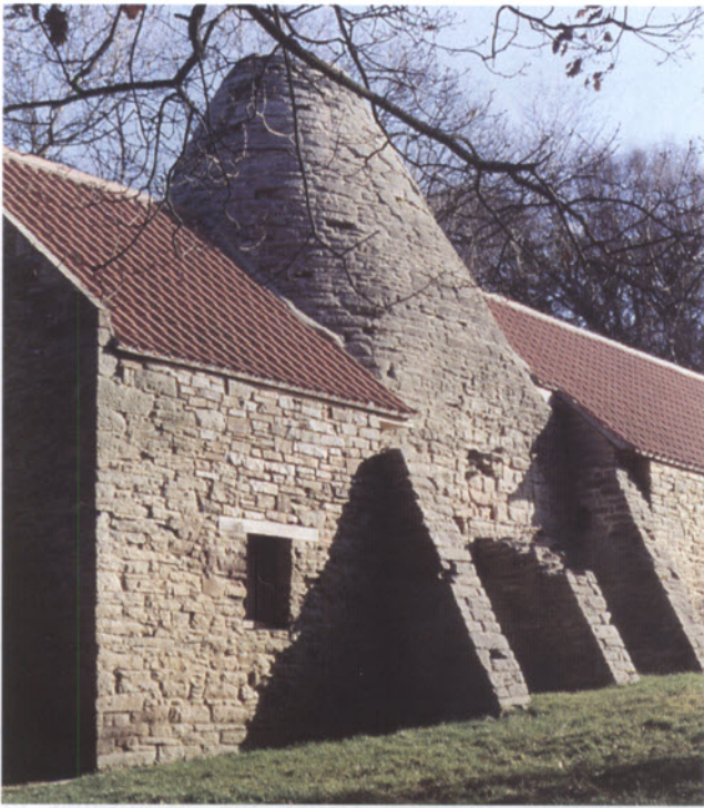
Figure 86: The early-18th-century cementation furnace at Derwentcote, Co Durham, with attached working buildings.
