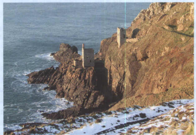
Figure 11: The Crowns engine house, Botallack mine, Cornwall, is set at the foot of a cliff on an outcrop of a rich tin and copper lode. This mine was worked from at least the 16th century.
