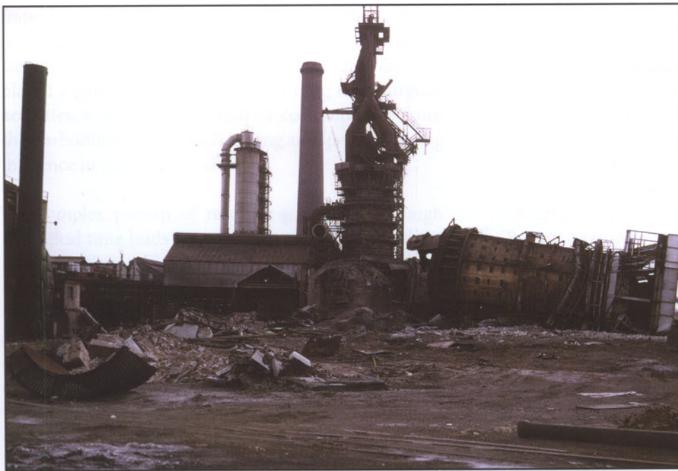
Figure 1: The blast furnaces at Stanton, Derbyshire, being demolished in 1976.
