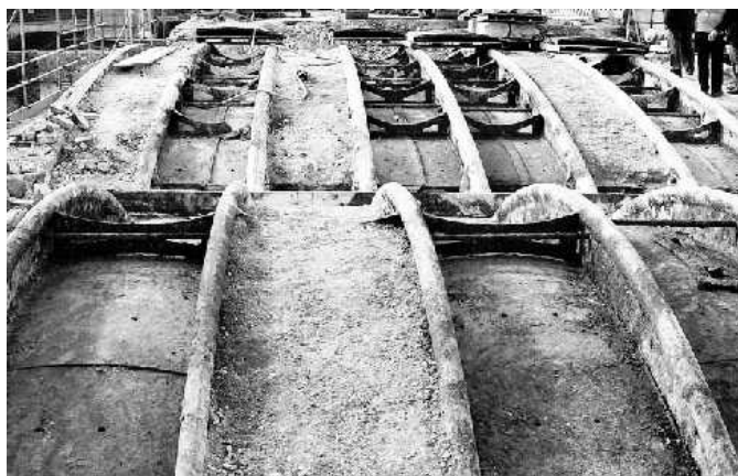
Brunel's Bridge as revealed when the later bricks were removed.
