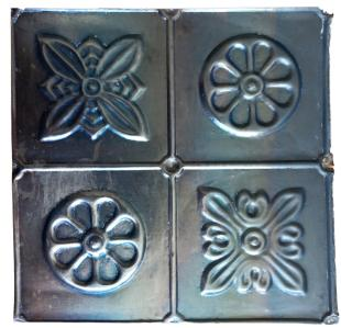
Figure 2: An example of an unpainted steel ceiling tile. Pin holes are present to the edges from where it was fixed to wooden furring strips on the ceiling.
